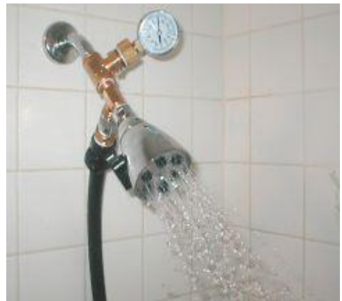
Here is the same shower immediately after flushing the toilet. Notice a substantial reduction in flow.
