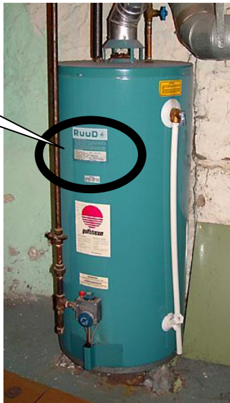
This is a hot water heater
