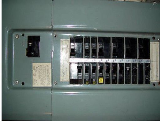
A Circuit Breaker Panel
